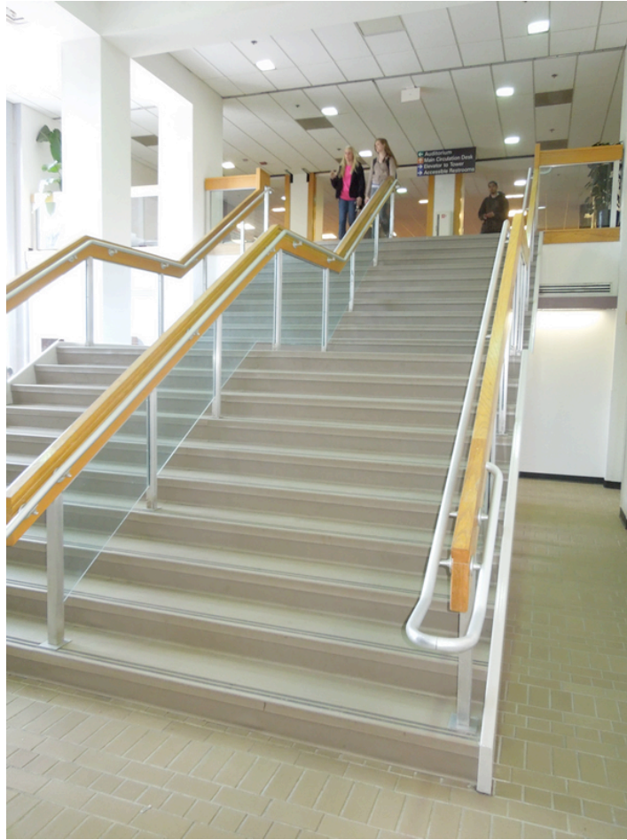
Figure 4 Appearance of the fully rebuilt stairs in the D. H. Hill Library (from bottom). Photo by author.
