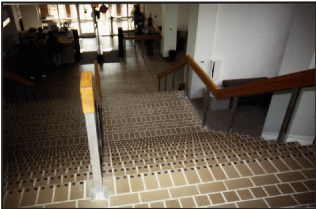
Figure 2 Appearance of the modified stairs in the D. H. Hill Library (from above). Photo by author.
