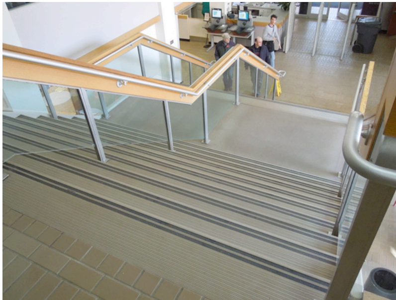
Figure 3 Appearance of the fully rebuilt stairs in the D. H. Hill Library (from above). Photo by author.
